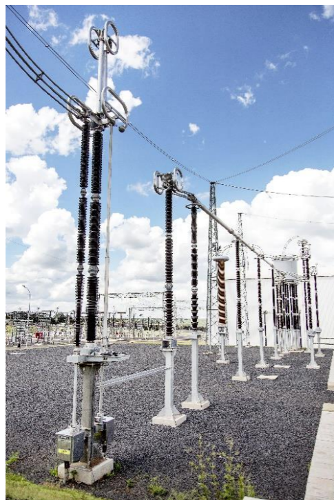
Plate 5.10 – Typical HVAC Disconnector Image: ©ABB
