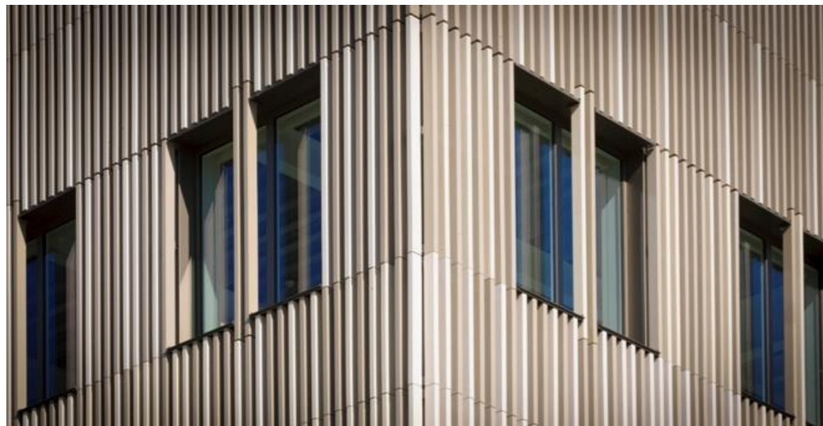
Plate 4.9 – Indicative illustrations of “baguettes”, showing shadowing effects to provide a layered texture to the facades
