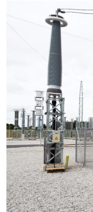
Plate 5.6 – Typical 400kV Cable Terminations Image: ©GE
