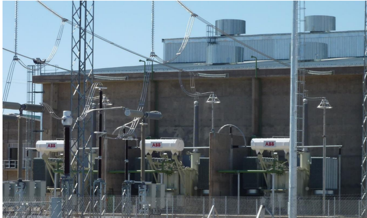
Plate 5.14 – Typical Interface transformers Image: ©ABB
