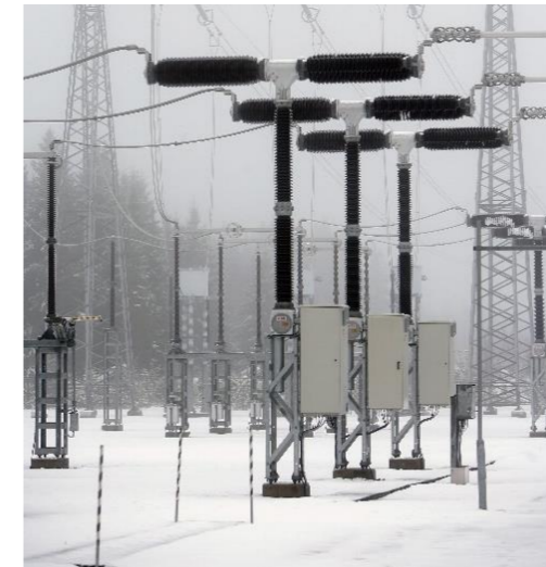
Plate 5.9 – Typical HVAC Circuit Breaker Image: ©ABB
